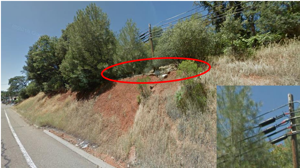
Figure 2. Paving Remnants as Seen From Placerville Drive (Source: Google Maps)
